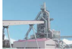
Wakayama Steel Works New No.1 blast furnace
