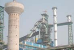
India: Bhushan Steel's steel works
