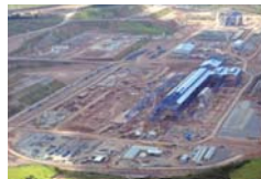
Construction site of integrated seamless pipe manufacturing works in Brazil
